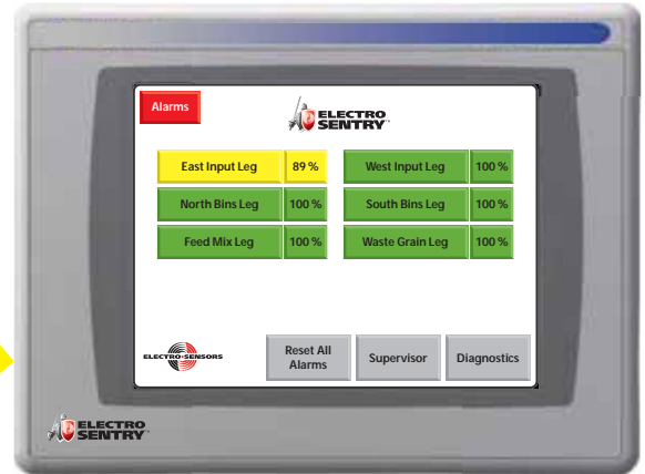
Alarm Condition on East Input Leg Plant Location Alarm View
