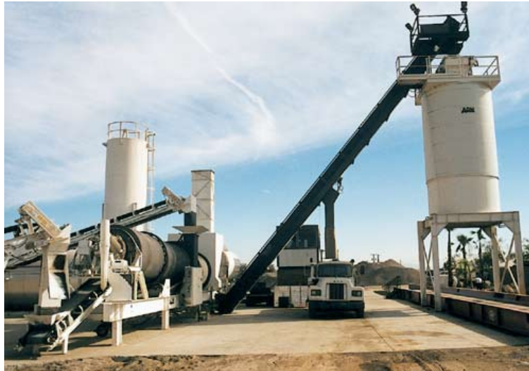
Asphalt Plant with pump mixer
