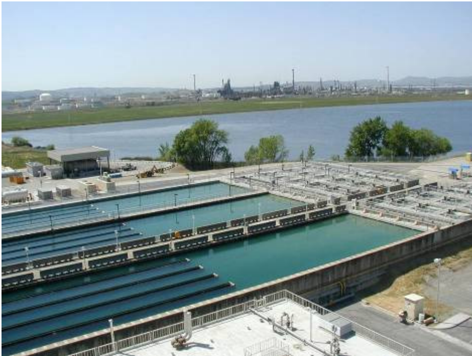
Waste Water Treatment Plant
