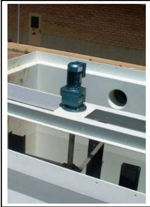
Vertical Flocculator Shaft & Motor
