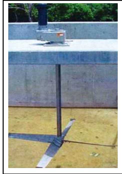
Vertical Flocculator Shaft & Motor
