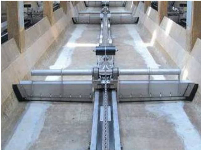
Clarifier Tank – Sludge Removal – Chain & Flight Drags
