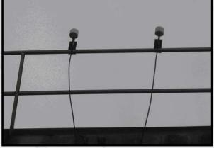
Two panel antennas mounted to RAM brackets.
