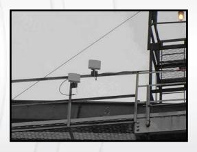
Two omni antennas using antenna hardware
